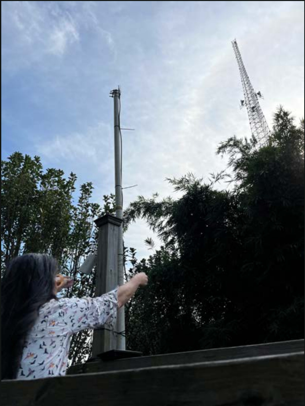
Caption IMG_7067: Installing an antenna for a network range test at a community farm in New Orleans.
