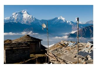
the villages use wireless Ethernet (802.11b/g standard) radios at 2.4 GHz from various manufacturers. The Motorola devices were used for the backbone connection due to their high reliability and robustness and to avoid signal interference. However, 802.11b/g radios were used for
